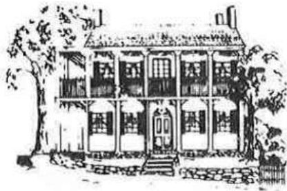
Phoenix House c.
