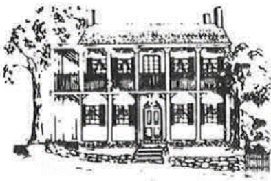
Phoenix House c. 1820
