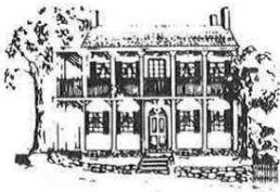
Phoenix House c. 1820
