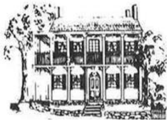
Phoenix House c. 1820
