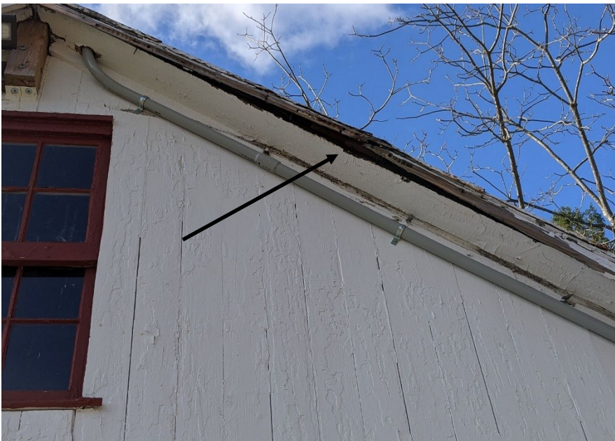
Photo E-6. View showing wood rot and loss at the rake board and soffit at the east elevation.
