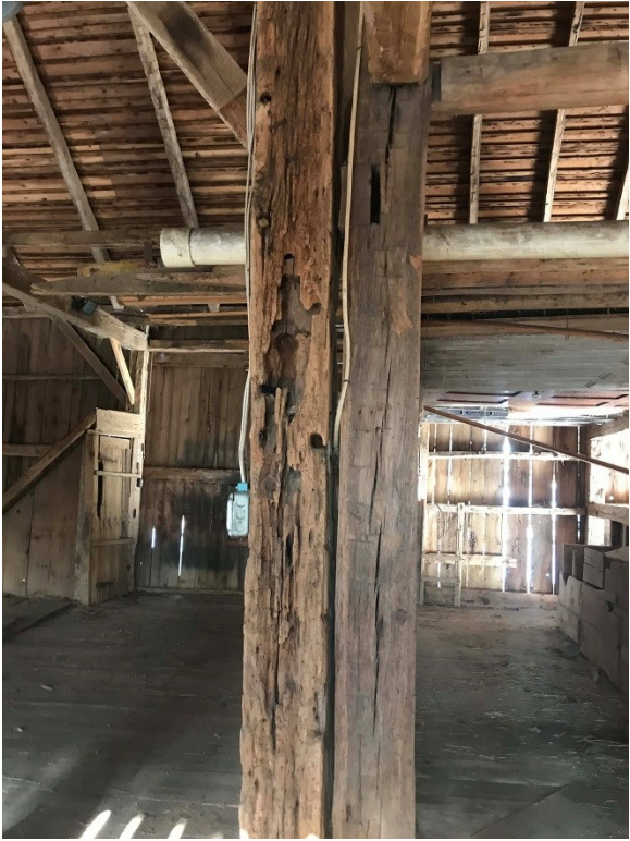
Photo I-17. View showing significant water damage at a post in Room 101.
