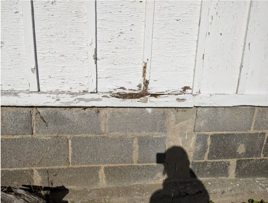
Photo E-7. View showing loss at the skirt board at the south elevation. Also note the vertical seam in the foundation below.
