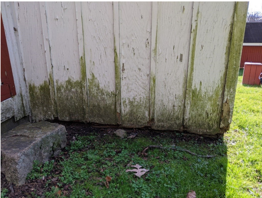
Photo E-10. View looking south at the shed extension showing significant biological growth and loss at the base of the siding.
