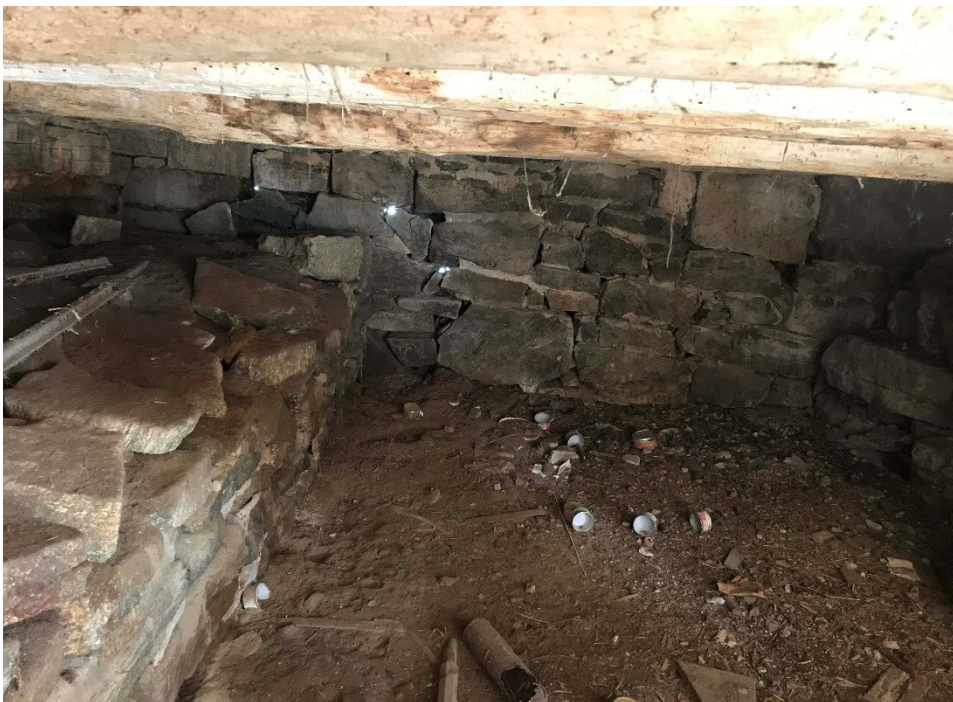
Photo I-10. View of the crawlspace showing mortar loss at the east foundation wall. Also note the debris on the dirt floor.
