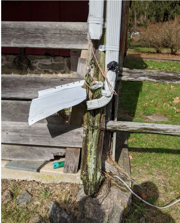
Photo E-9. View of the wood post at the southeast corner, which exhibits significant loss and biological growth due to the position of the adjacent leader.
