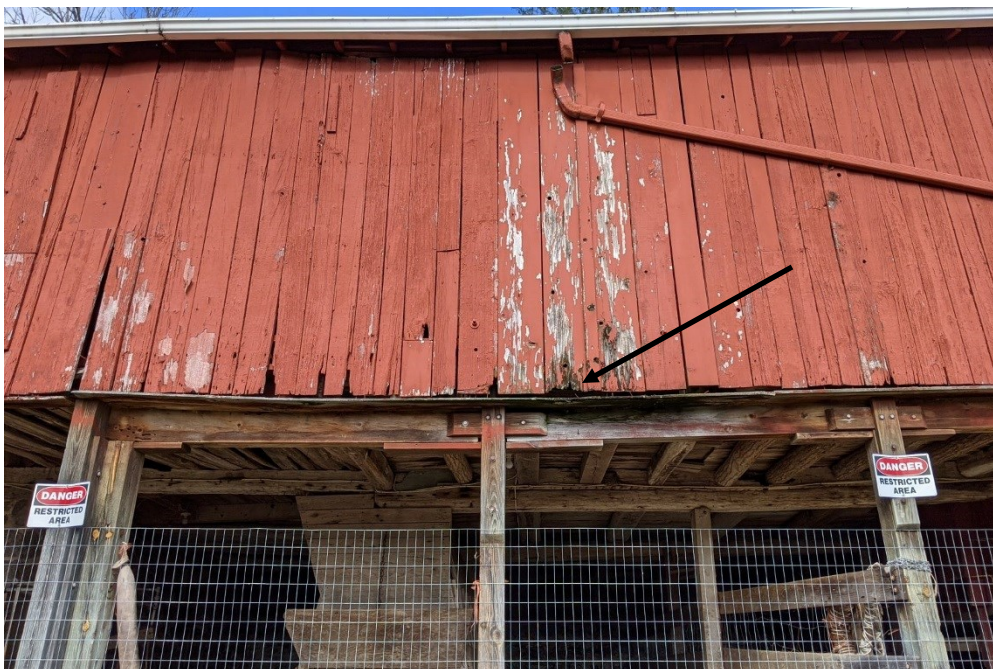
Photo E-10. View of the south elevation showing significant paint loss and wood rot at the siding caused by the disconnected leader above. Also note the projecting floor board, which has pulled away from the ends of the siding.
