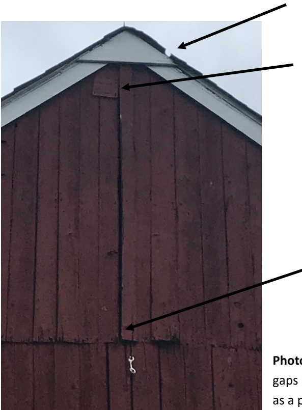
Photo E-11. Detail view of the bottom edges of siding boards at the west elevation showing wood loss, splits, and paint loss.
