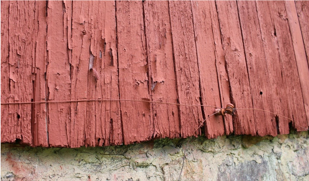
Photo E-11. Detail view of the bottom edges of siding boards at the west elevation showing wood loss, splits, and paint loss.
