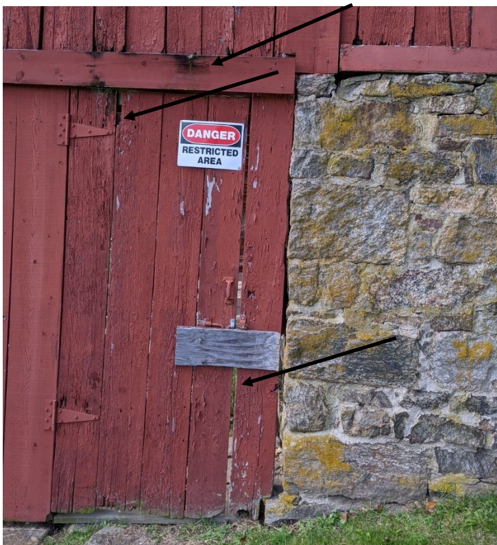
Photo E-8. View of door D102 at the east elevation showing wood loss, paint loss, and separation between boards. Also note the wood rot at the door hood above, and the loss at the ends of the siding boards.
