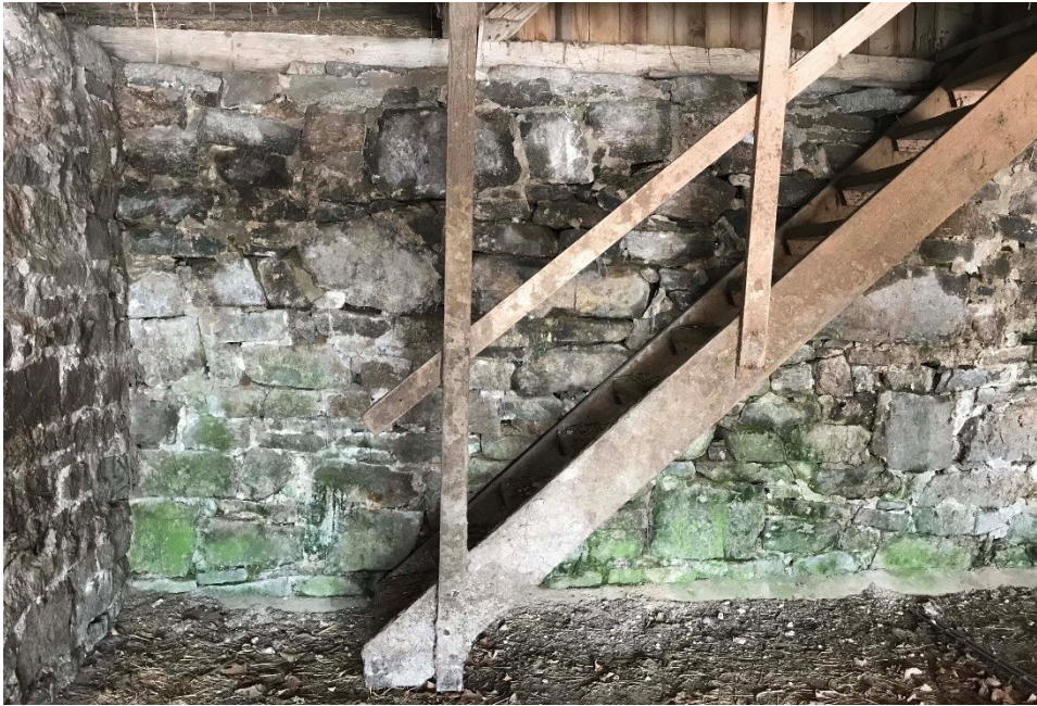
Photo I-11. View showing mortar loss and biological growth at the north foundation wall in Room 001.
