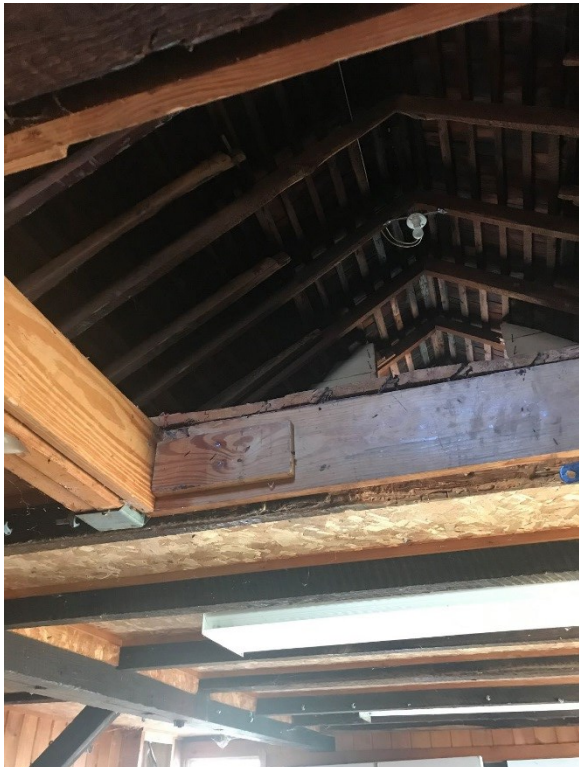
Photo I-4. View looking up at the attic showing earlier framing incorporated with the roof framing.
