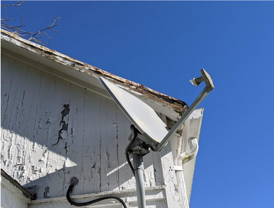
Photo E-9. View showing wood rot and loss at the rake board at the west elevation. Also note the paint failure at the siding.
