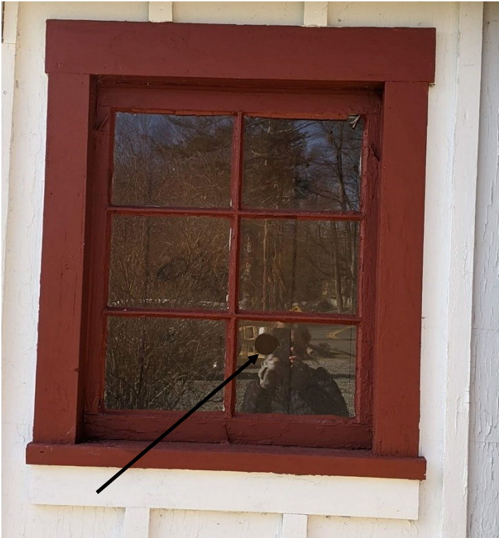
Photo E-5. View of window W102 showing a hole in the bottom right pane.
