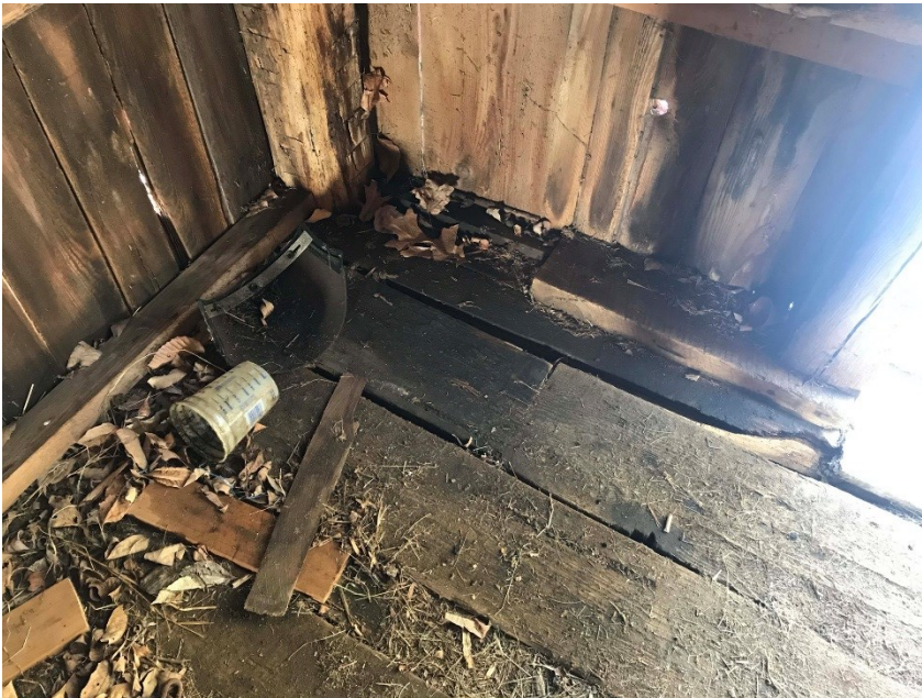
Photo I-18. View showing wood rot and moisture damage at the northwest corner of Room 102.
