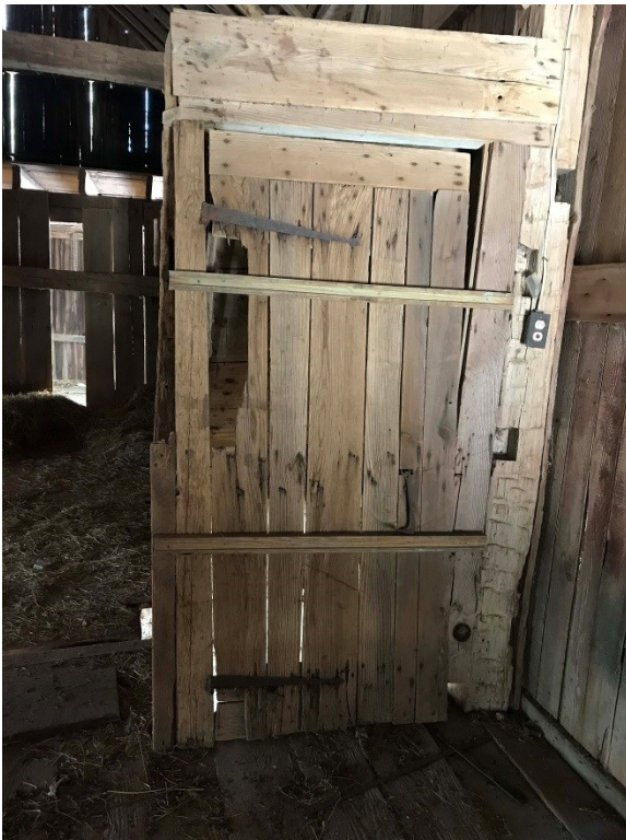
Photo I-14. View of door D110 showing wholesale loss at one board, gaps between boards, and displacement within the opening.
