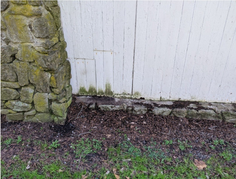
Photo E-11. View showing biological growth and loss at the base of the wood siding adjacent to the chimney. Also note the mortar loss and biological growth at the chimney.
