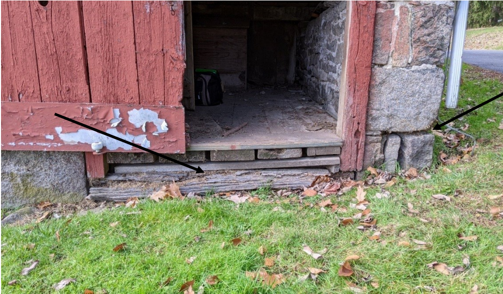
Photo E-7. View of the mismatched infill below door D102. Also note the mortar loss at the corner of the foundation and the paint loss at the door.
