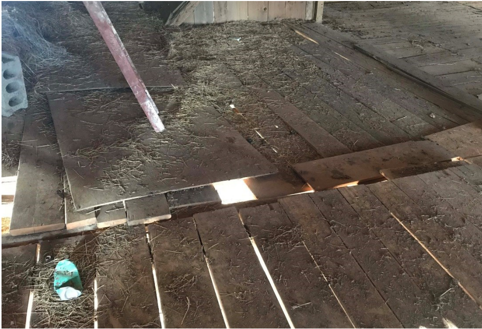
Photo I-15. View showing loss and unevenness at the floor.
