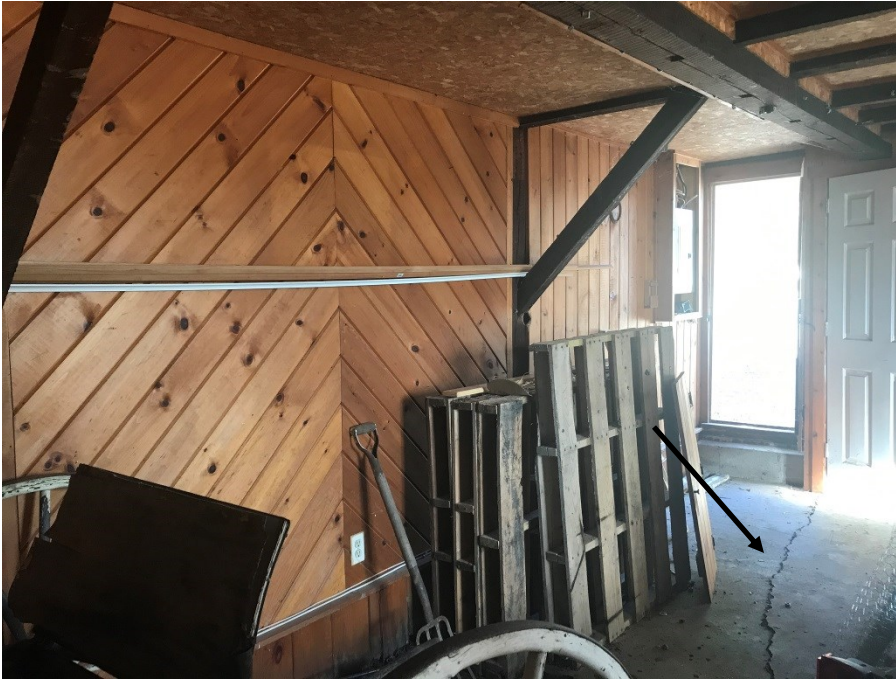
Photo I-5. View showing a significant crack in the concrete floor.
