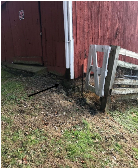
Photo E-6. View of the cut-off leader at the northwest corner and the related wood rot and biological growth.
