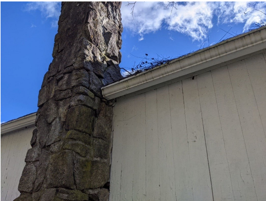
Photo E-12. View showing debris at the gutter adjacent to the chimney.
