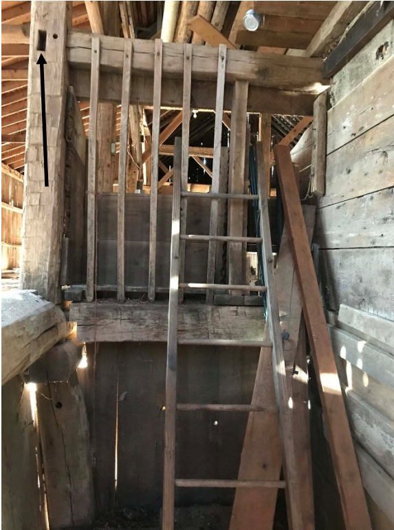
Photo I-13. View looking west in Room G003 showing loss of a horizontal beam at the enclosure.
