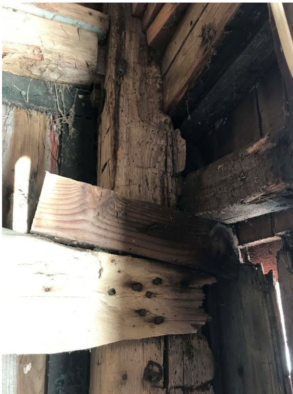
Photo I-12. View showing wood rot and loss at the northeast corner post in Room G001.
