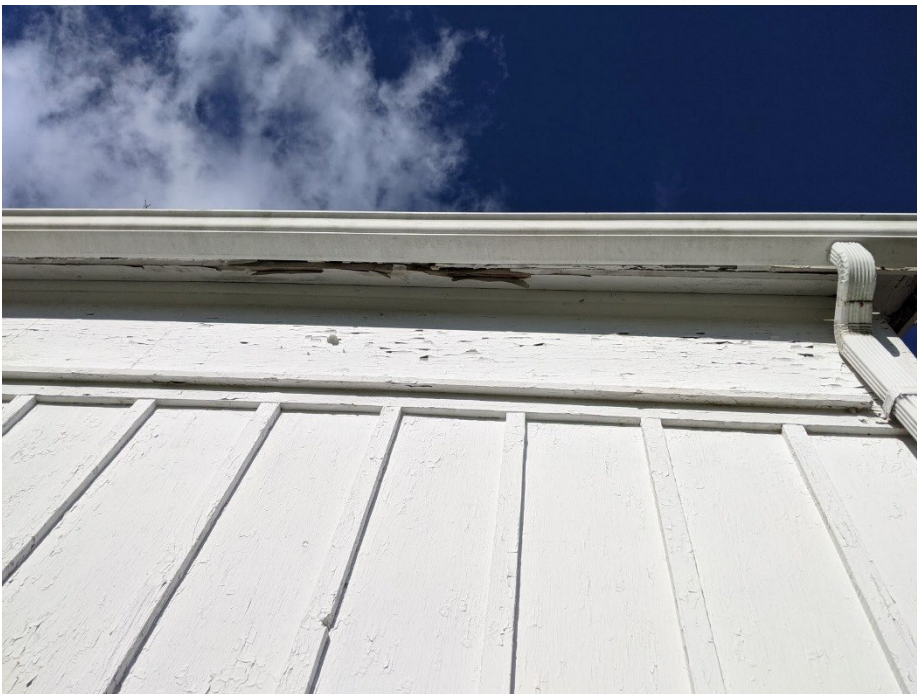
Photo E-8. View of the soffit showing wood rot.
