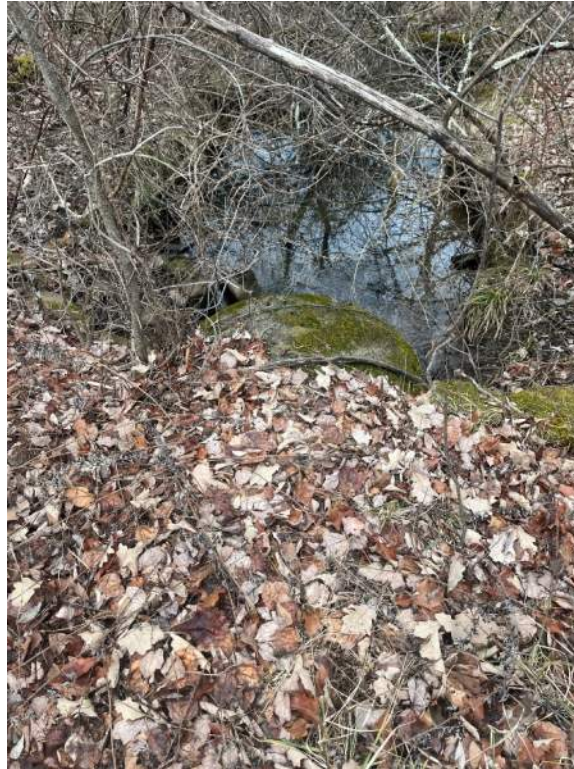
Culvert under Patriot's Path Downstream of Property
