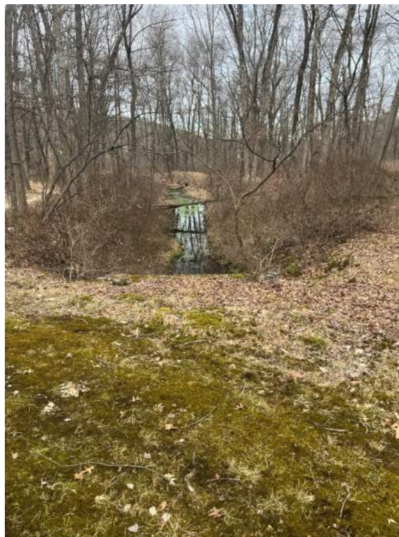
Outfall and Stream off of Dean Road
