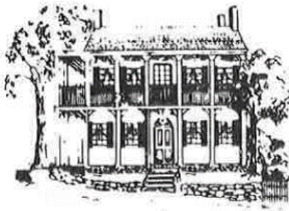
Phoenix House c. 1820
