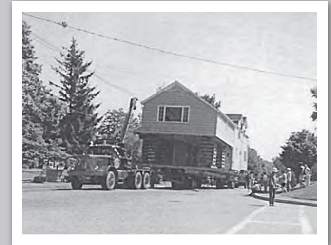
On July 7, 1977, the best show in town was watching the Freeman Ayers' "new" house move from the site of the new post office to 50 Main Street. After obtaining permission from the government, Mr. Freeman saved the Ayers home from demolition. Mendham Borough Library archives
