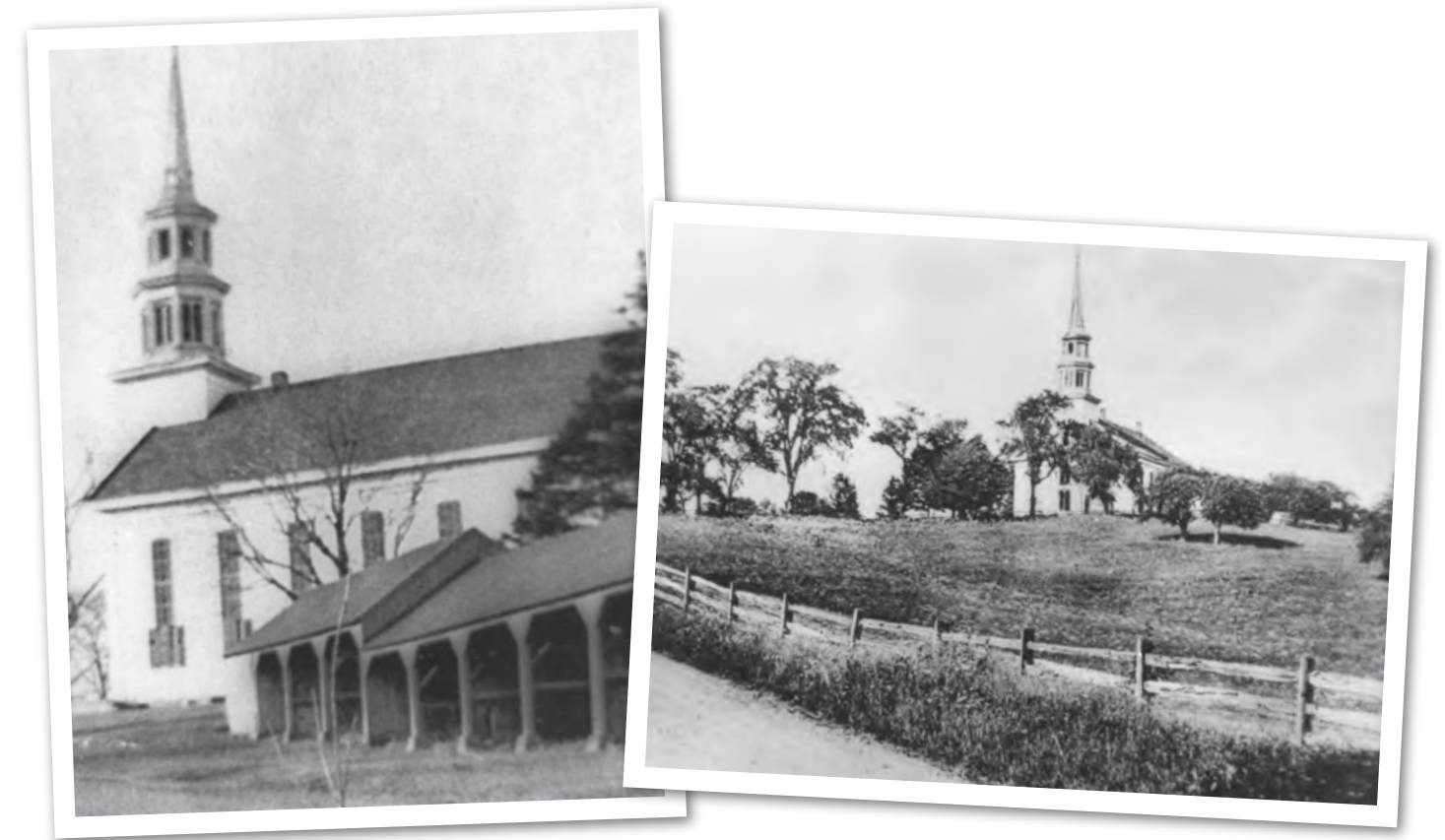
Left: The Hilltop Church stables before they were destroyed by fire.
