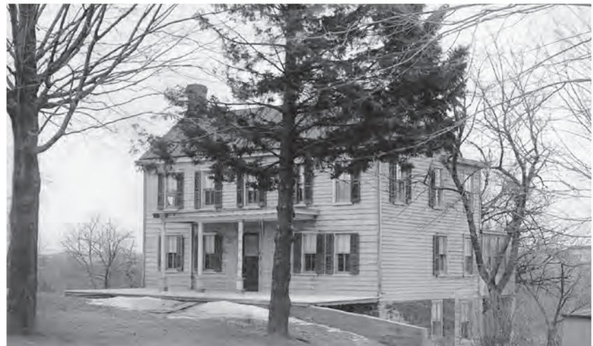
Sharkey House—formerly Restformi, for a time a retirement home for telephone workers—sits on East Main Street streams that become the Raritan and Passaic Rivers. Courtesy of Don Preziosi
