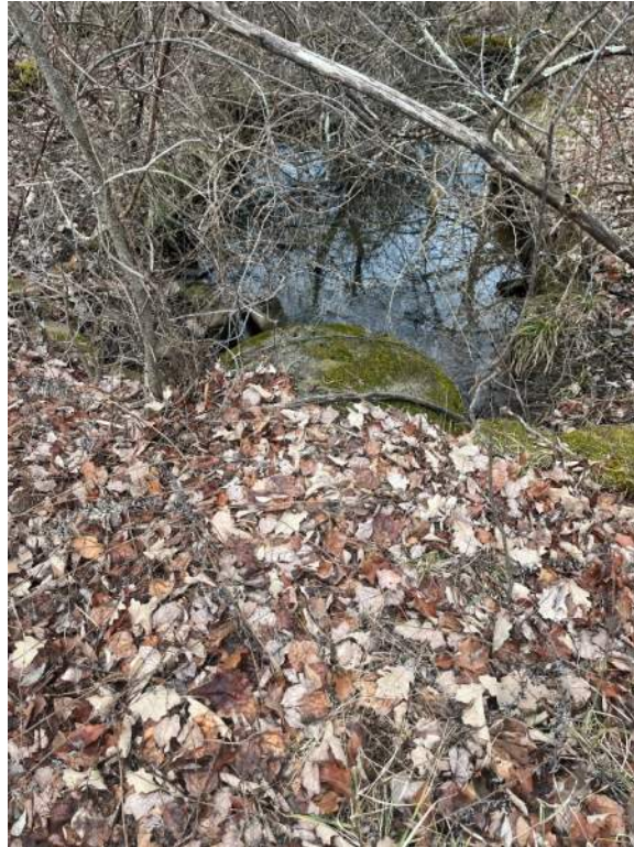
Culvert under Patriot's Path Downstream of Property
