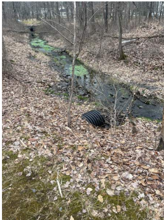
Interconnection Pipe Downstream of Dean Road Outfall
