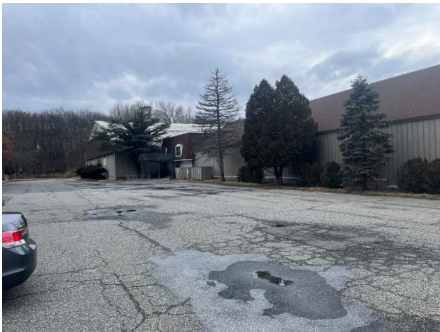
Existing Building with Adjacent Trees
