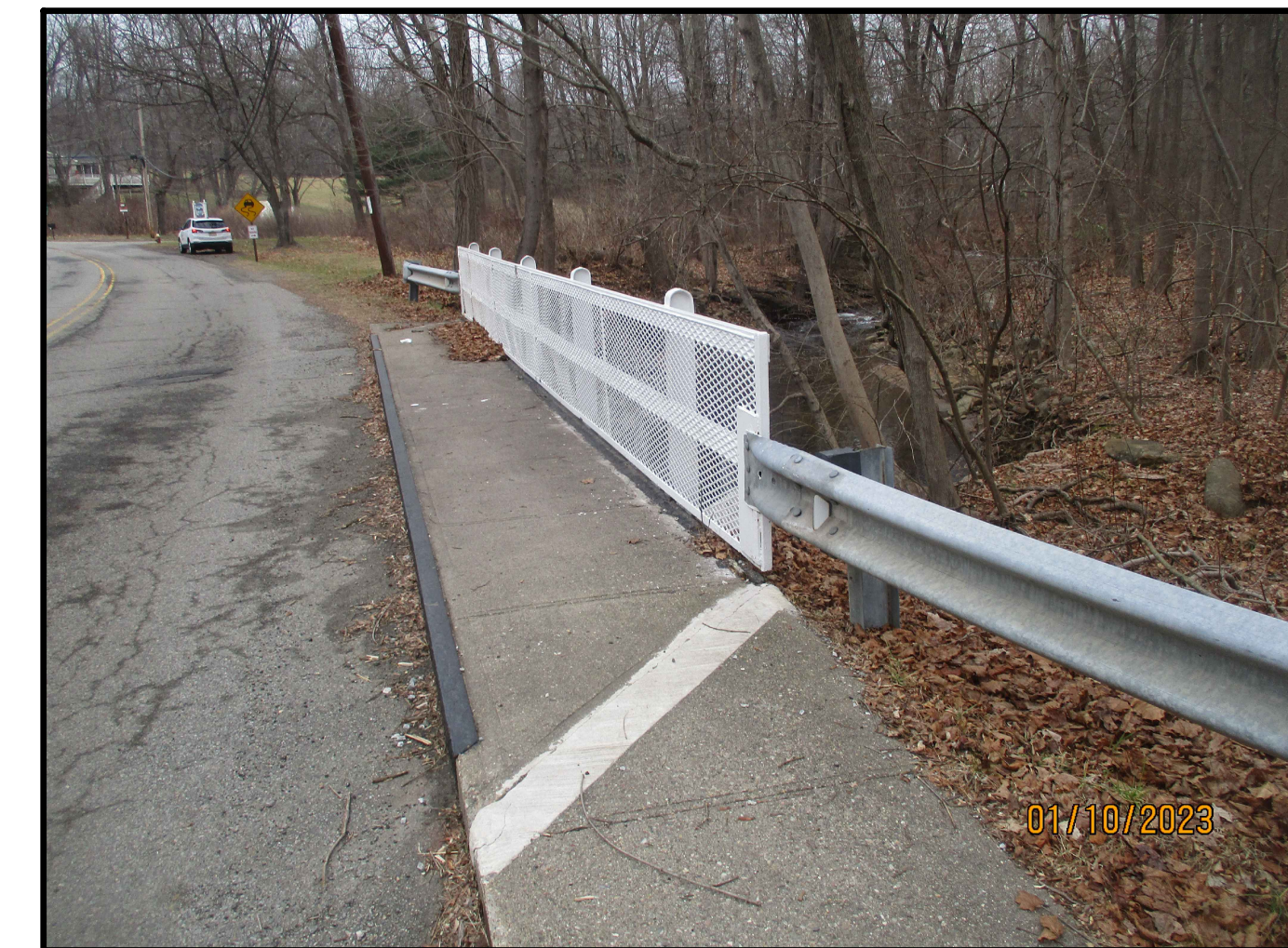
CONCRETE SIDEWALK AND STEEL CHANNEL RAILING WITH STEEL LATTICE LOOKING NORTHEAST
