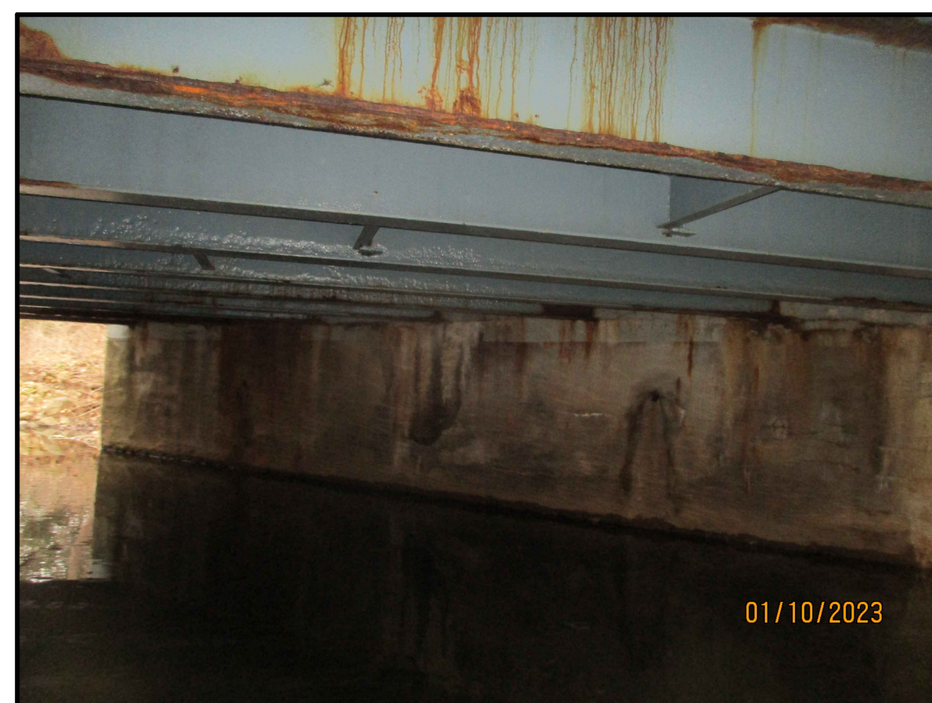
STEEL BEAMS AND CONCRETE ABUTMENT LOOKING UNDERSIDE OF BRIDGE DECK/ROADWAY
