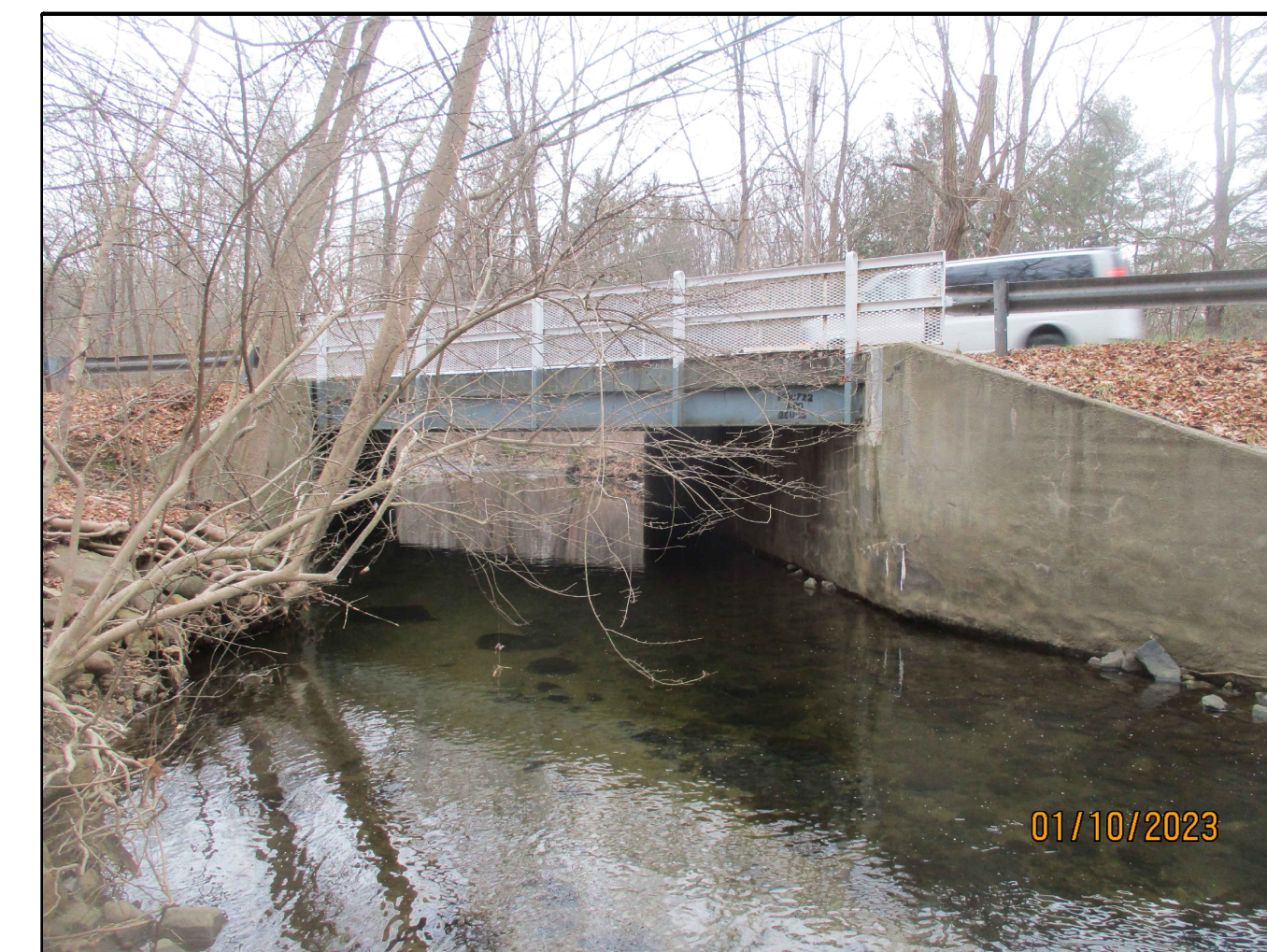
EAST FASCIA (UPSTREAM FACE) LOOKING DOWNSTREAM
