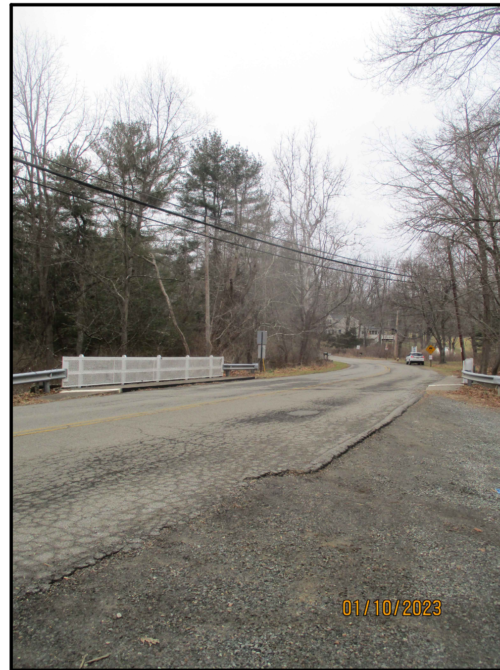
SOUTH APPROACH LOOKING NORTHWEST
