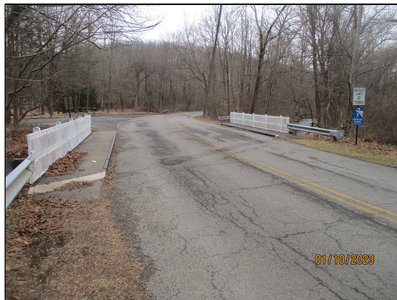
NORTH APPROACH LOOKING SOUTH
