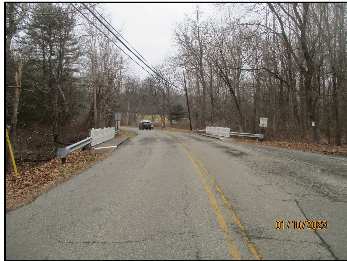
SOUTH APPROACH LOOKING NORTH
