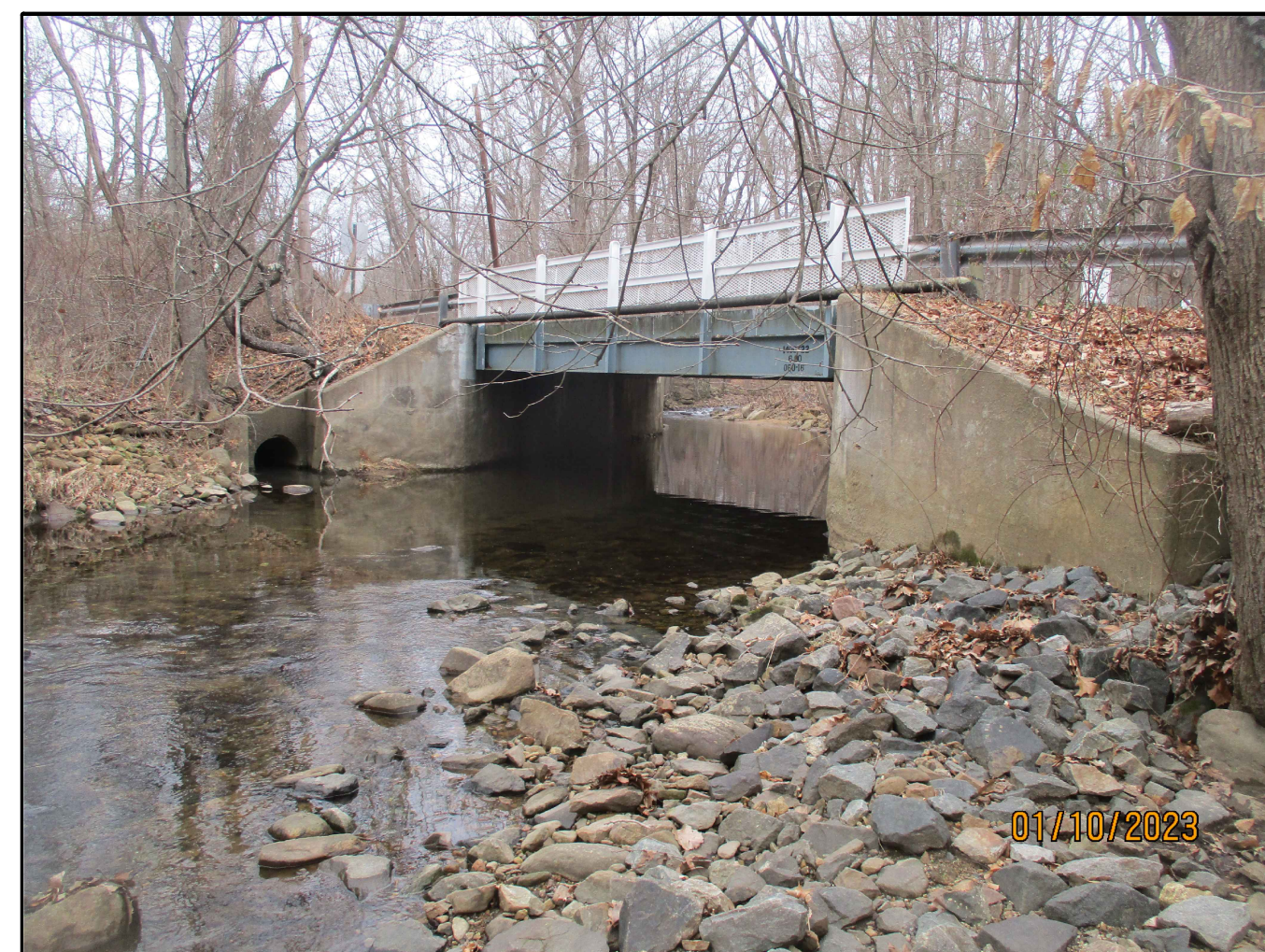
WEST FASCIA (DOWNSTREAM FACE) LOOKING UPSTREAM
