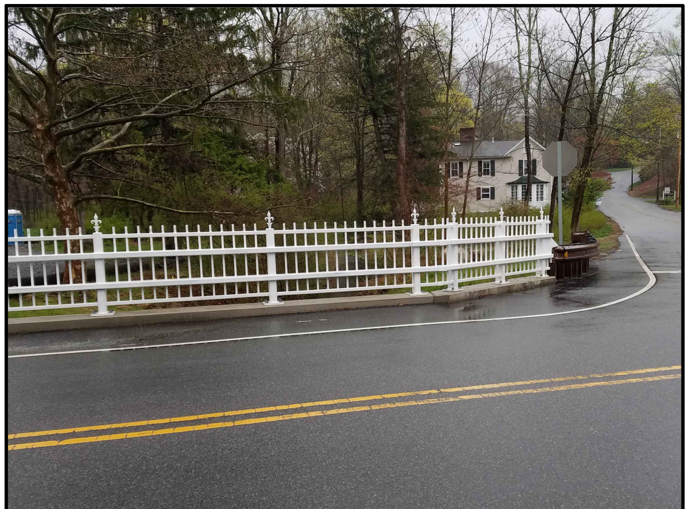
ORNAMENTAL 4-RAIL ASSEMBLY BRIDGE RAILING
