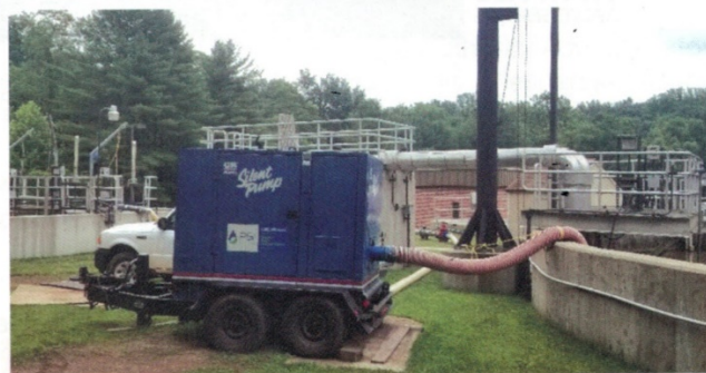
Figure 4: MLR bypass pump provided by Pumping Services with orange suction line adjacent to MLR pumps, and yellow discharge line leading to anoxic tank on left.
